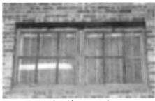
Figure 58. Paired steel hopper windows over former freight door at north end of east elevation
