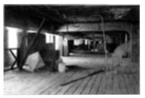
Figure 38. View of the mezzanine looking north. Floor boards were reused from demolished first floor structure in 1970
