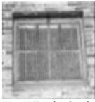
Figure 59. Typical single steel hopper, approximately 3' square window in main warehouse
