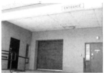
Figure 77. Pressed metal ceiling panels at underside of north loading dock canopy
