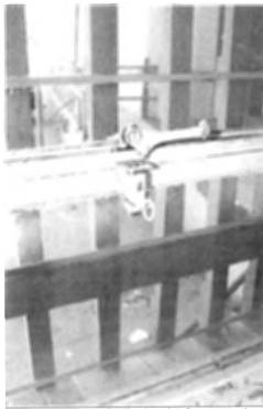
Figure 74. Typical window latching hardware at steel office windows
