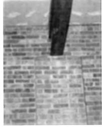
Figure 71. Interior detail of masonry exterior wall showing what appears to be repointing
