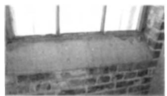
Figure 72. Cement wash at window sills applied over bottom rail preventing window from opening
