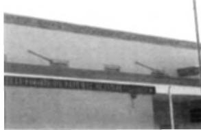
Figure 80. Loading dock canopy with tension rods and turnbuckles and portion of sign from the State Archives era
